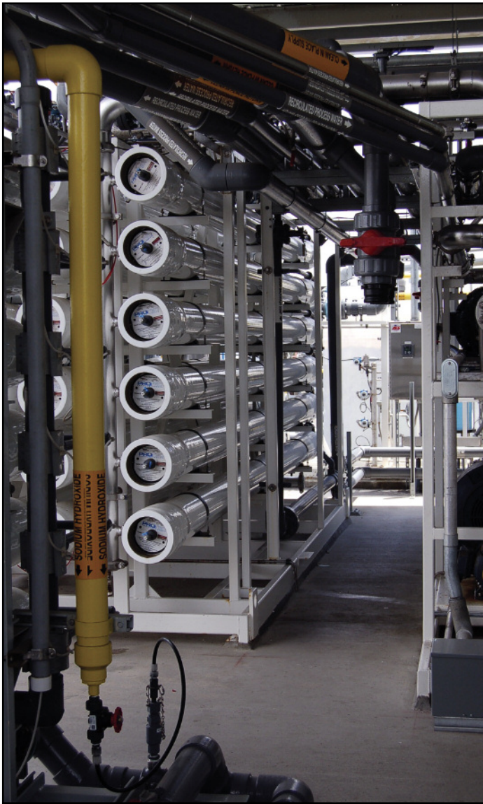
Long Beach Water's experimental research facility produces 300,000 gallons of fresh desalinated water each day.
