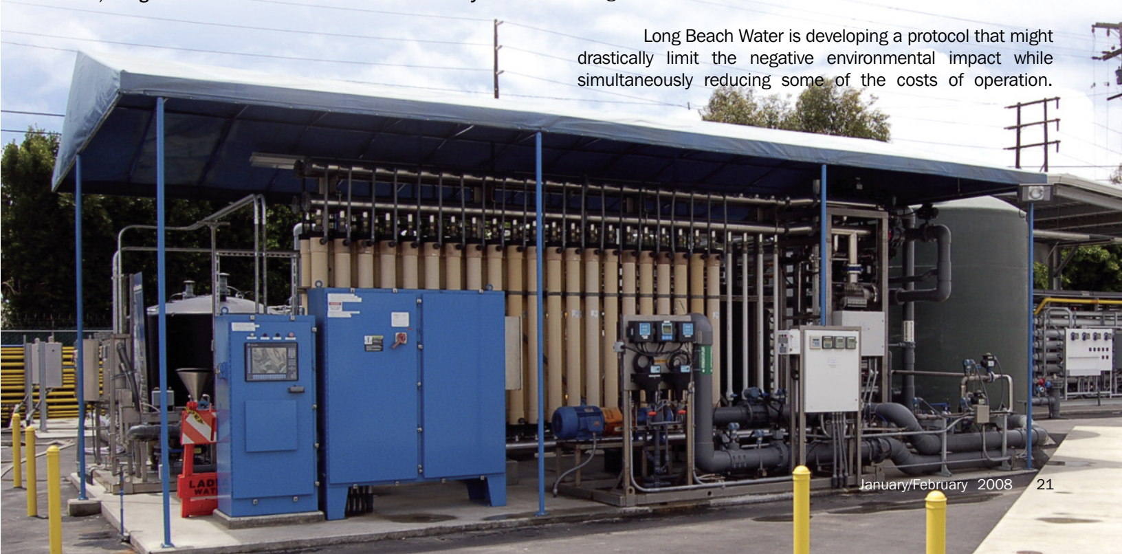
Long Beach Water's experimental research facility produces 300,000 gallons of fresh desalinated water each day.
