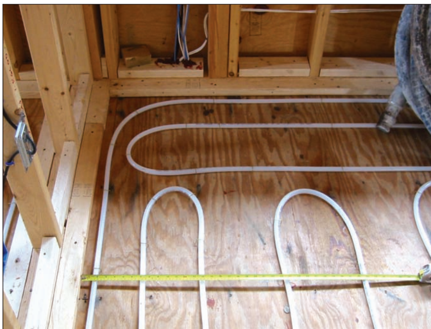
Above: Plastic tubing is laid at precise measurements on the subfloor.
