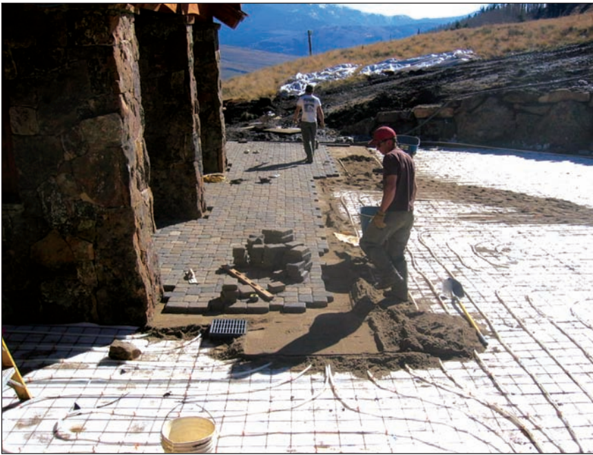
Above: Workers installing pavers over a Hydronic snow melting system.
