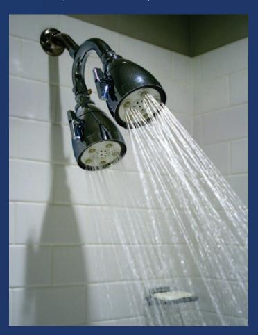
Showerheads must also be equipped with an automatic compensating valve that complies with ASSE 1016 or ASME A112.18.1/CSA B125.1 and be specifically designed to provide thermal shock and scald protection at the flow rate specified above.
