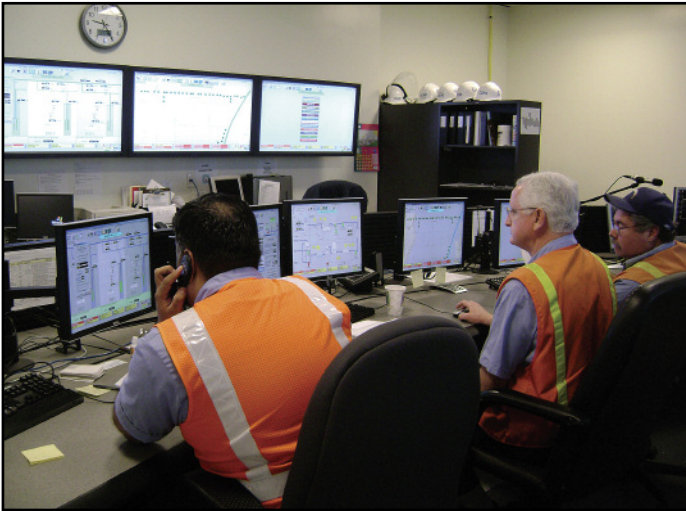
OCGRS workers monitor the filtration process from the control room of the Fountain Valley, Calif. facility.
